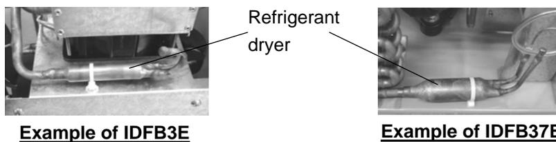
The refrigerant dryer is packaged in moisture-proof packaging. If it is left unsealed, it will absorb moisture from the atmosphere and become unusable. After opening the packaging, mount it quickly (within a few minutes.)
